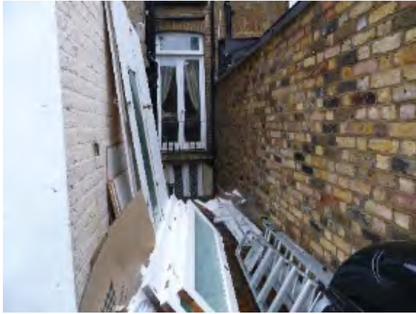
7. Discarded materials around rear
